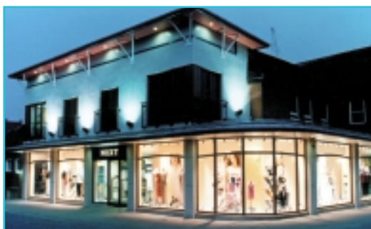
Delancey Estates, King Edward Court, Windsor Project Management, remodelling and refurbishment of centre.
