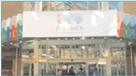
Norwich Union Milner Retail Partnership Pyramid Shopping Centre, Birkenhead Project Management, Quantity Surveying, Planning Supervision. Upgrading works - £1m.
