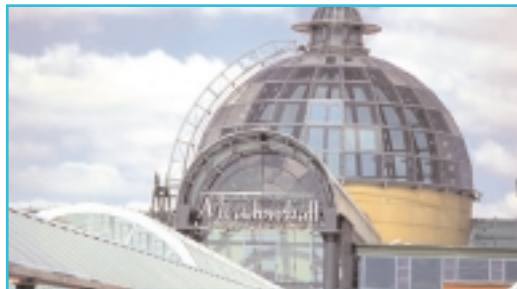
British Land Plc, Meadowhall Centre, Sheffield Pre-acquisition survey, Project Management of refurbishment works.
