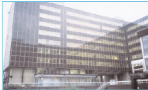
Entec UK, Northumbria House, Regents Centre, Gosforth, Newcastle-upon-Tyne Acquisition Building Survey, Contract Administration of internal refurbishment and external fabric repairs
