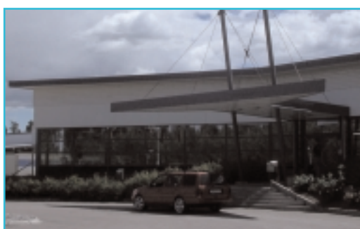
HSBC Private Bank plc Sweden Building survey of distribution warehouse
